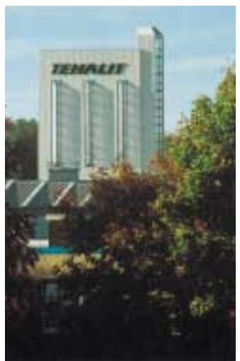
Tehalit headquarters in Heltersberg - Germany
